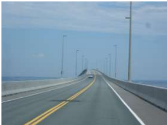
The Confederation Bridge approaching PEI
